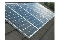
most popular are modules which can either sit on the roof or be integrated into it. The technology is most efficient when oriented due south. However panels orientated south of east or west are suitable. Generally panels orientated away from due south require a greater surface area to generate a set amount of energy.
